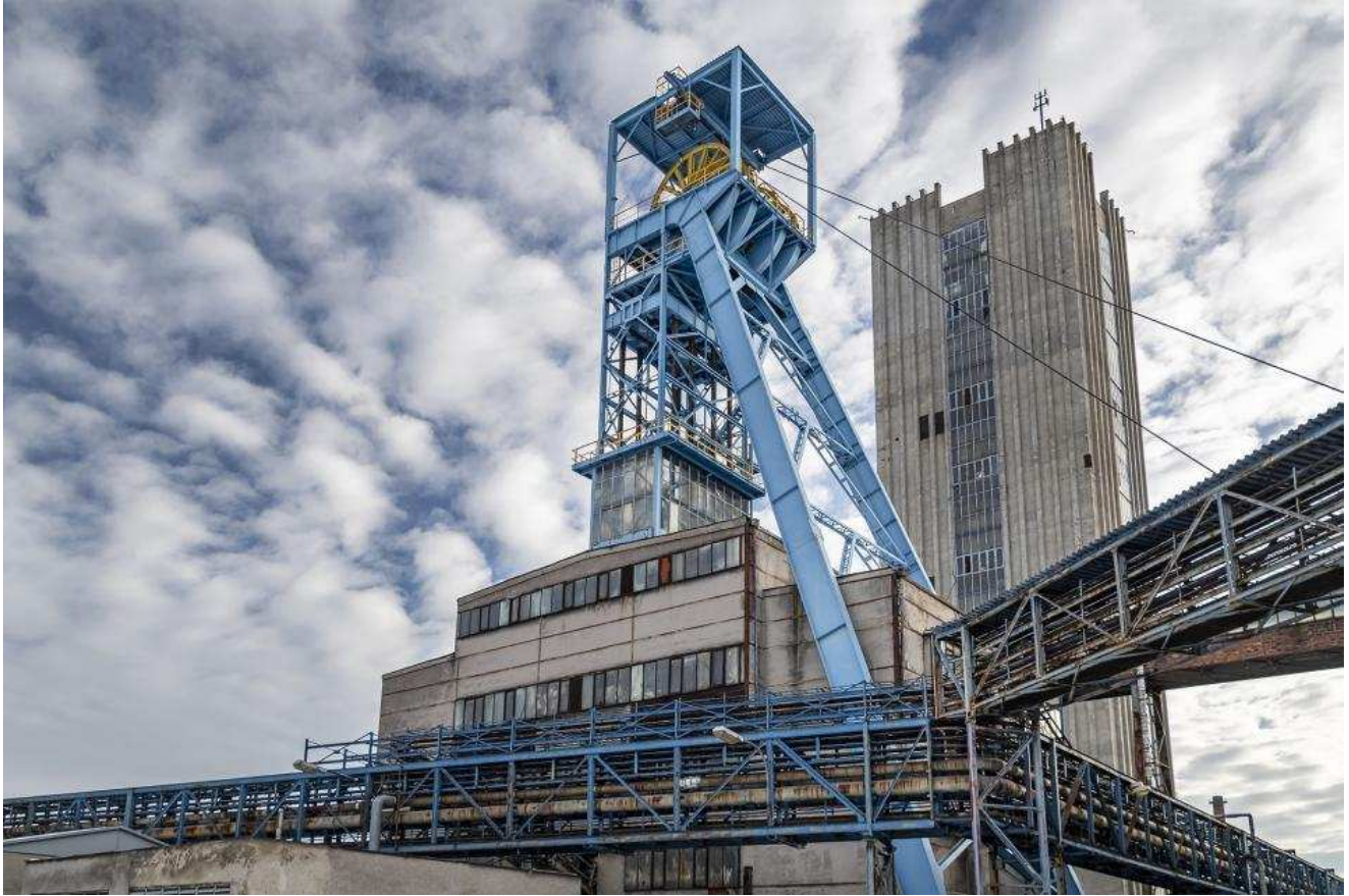
Figure 41: Shaft hoisting system at Darkov deep coal mine
