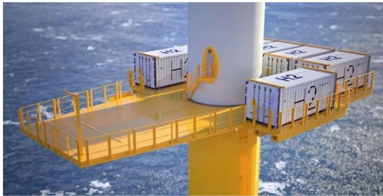
**Figure 4-7 - Turbine-integrated hydrogen production platform concept [Siemens Gamesa]**
