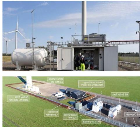
Figure 4-43: Brande Hydrogen Project
