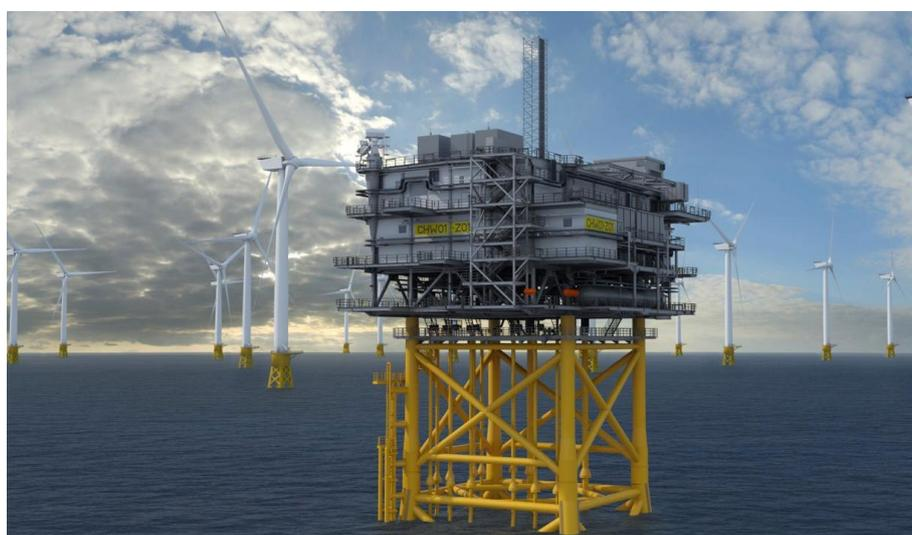
Figure 5-7: HVAC transformer platforms for Greater Changhua Offshore Wind Farms [11]
