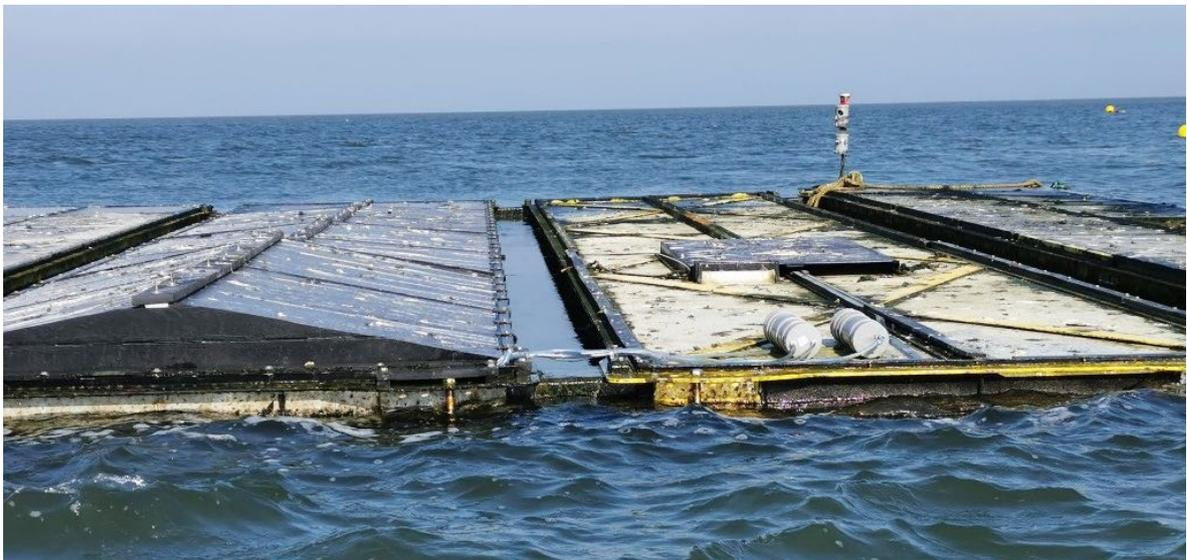
**Figure 4-51: Pilot project for floating solar by Oceans of Energy in the Dutch North Sea**
