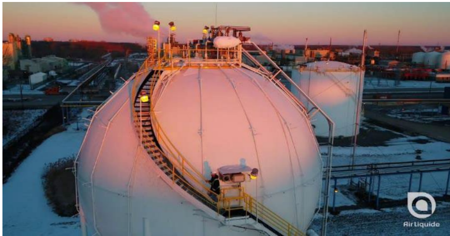
Figure 186: Air Liquide's PEM Electrolyser in Bécancour, Canada
