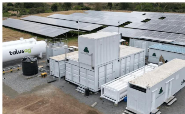
Figure 20: TalusAg installation in Kenya 56
