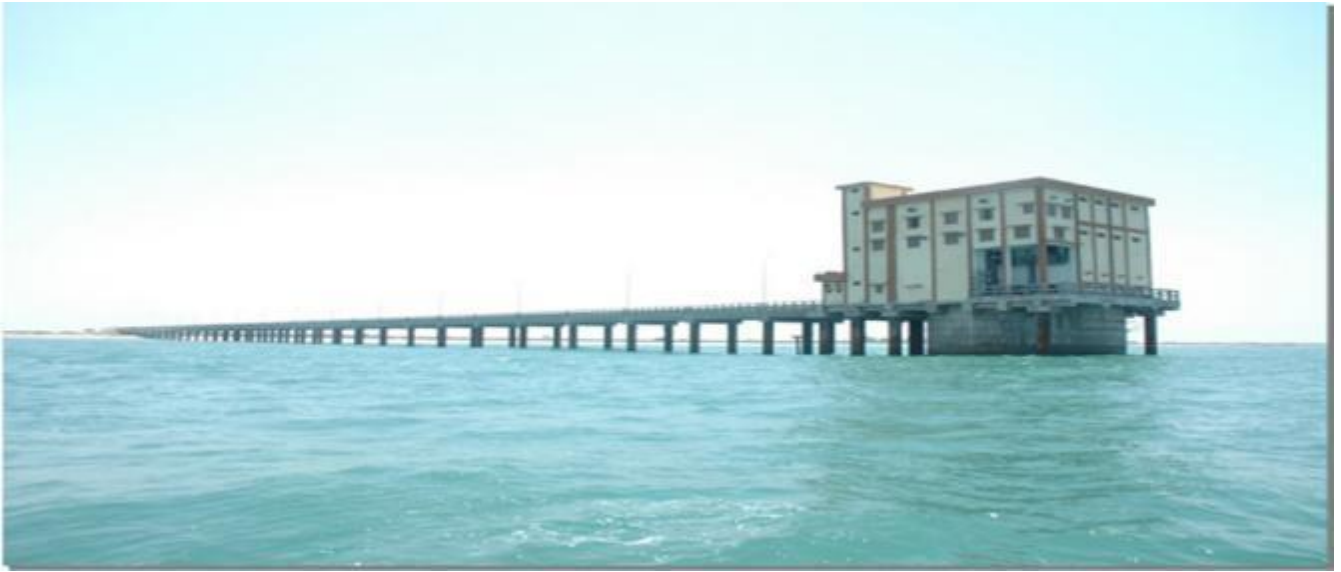
Figure 3-2 – Offshore Intake arrangement for 45 MLD (Million Litres per Day) Desalination Plant at CPCL, Chennai
