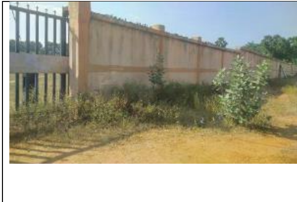
Figure 5-3- Green Hydrogen Hub Site – Main Gate
