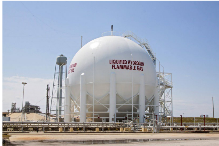
Figure 50: Hydrogen spherical storage (representative image)
