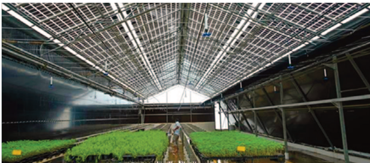
Greenhouse PV using Building Integrated Photovoltaic (BIPV) modules. © Jain Irrigation.
