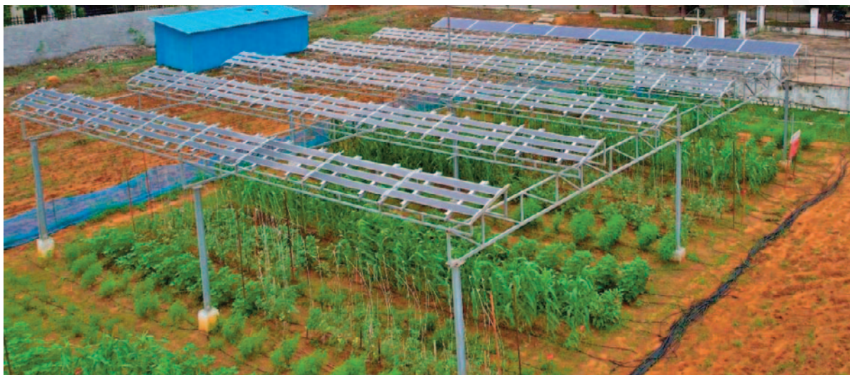
Semi-transparent PV panels installed at Seed Research and Technology Centre (SRTC), PJTSAU, Rajendranagar, Hyderabad. © Renkuba.
