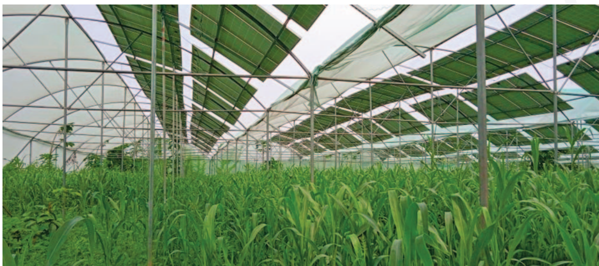
Plant B, Indra Solar Farm, Agrivoltaics plant, Tikamgarh, Madhya Pradesh. © Khare Energy Private Ltd.
