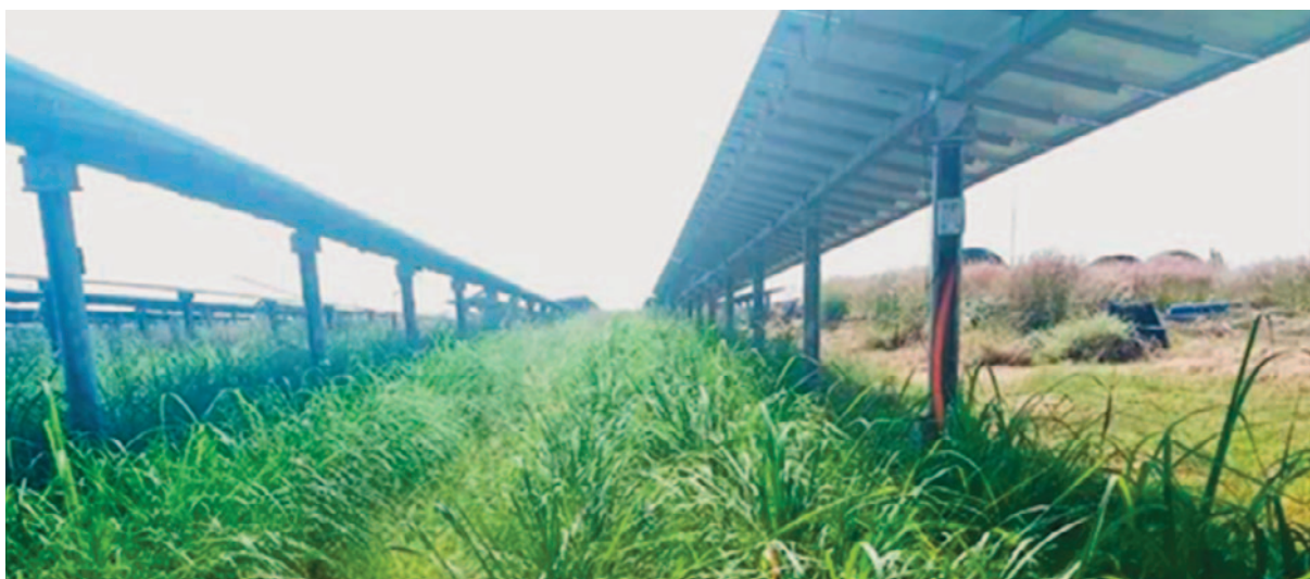
Mahindra Susten plant at Tandur with lemon grass. © Mahindra Susten.
