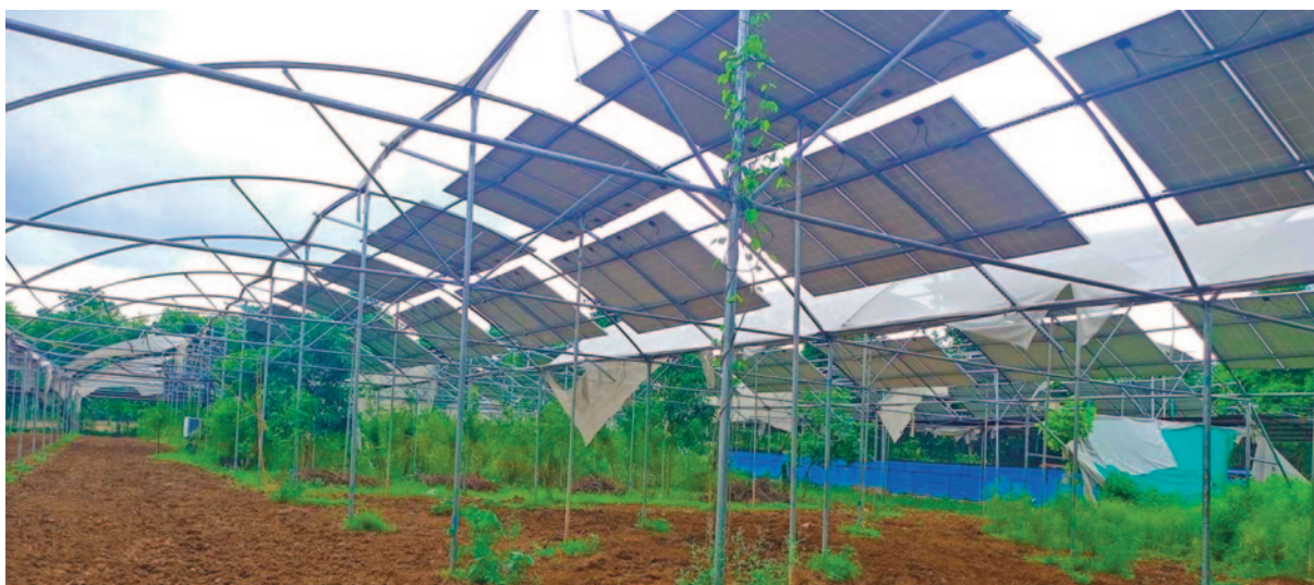
PV panels retrofitted onto a polyhouse. © Khare Energy Private Ltd.
