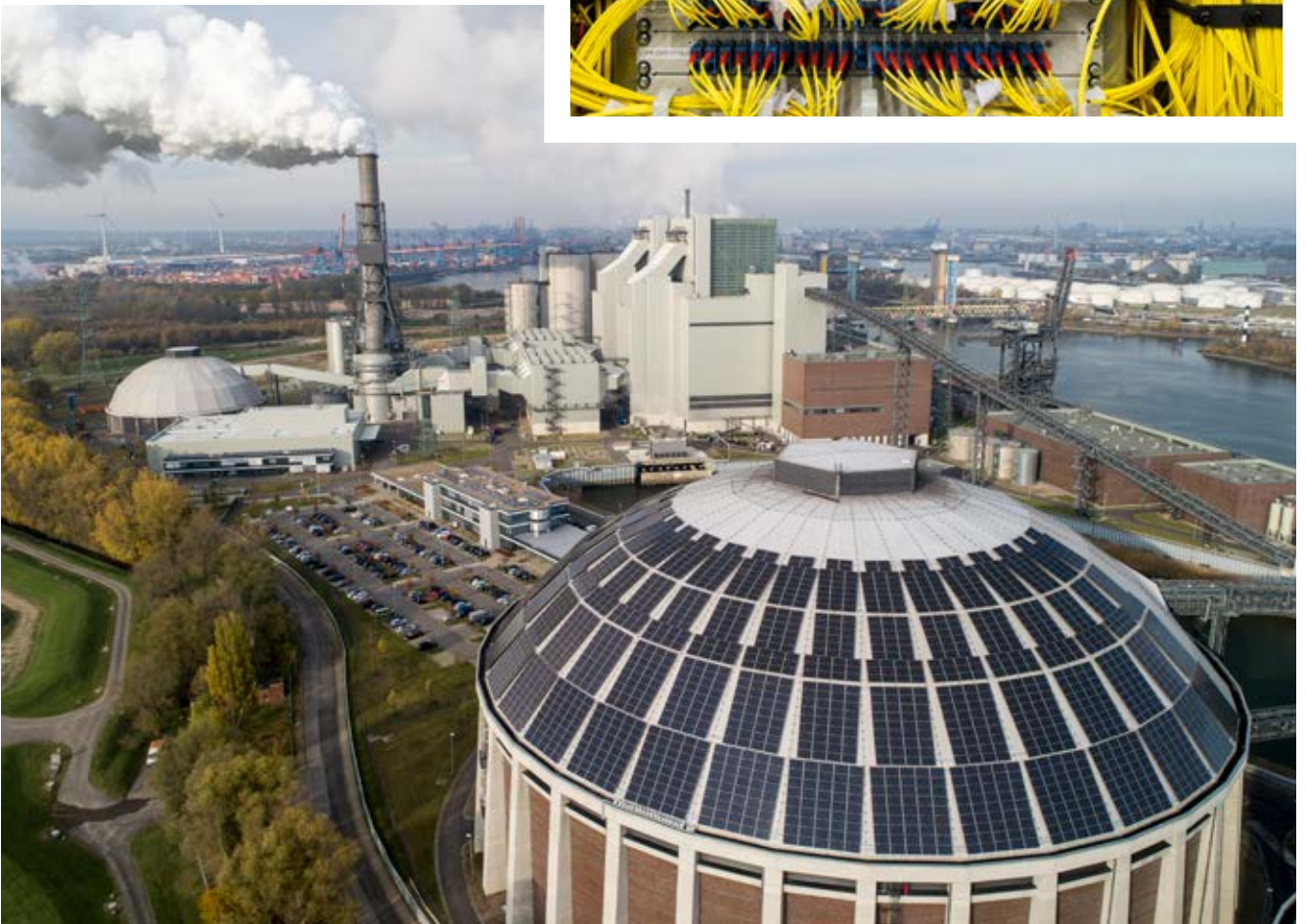
Reusing the old coal-fired power plants: Lignite and hard coal can be replaced by fuels such as biomass, gas and green hydrogen. Data centres will be set up at some sites. And the former coal sites (and part of the power plant site) can be used for solar or wind energy.
