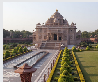
GIZ Installs PV Port Systems in Swaminarayan Akshardham Mandir, Gandhinagar
