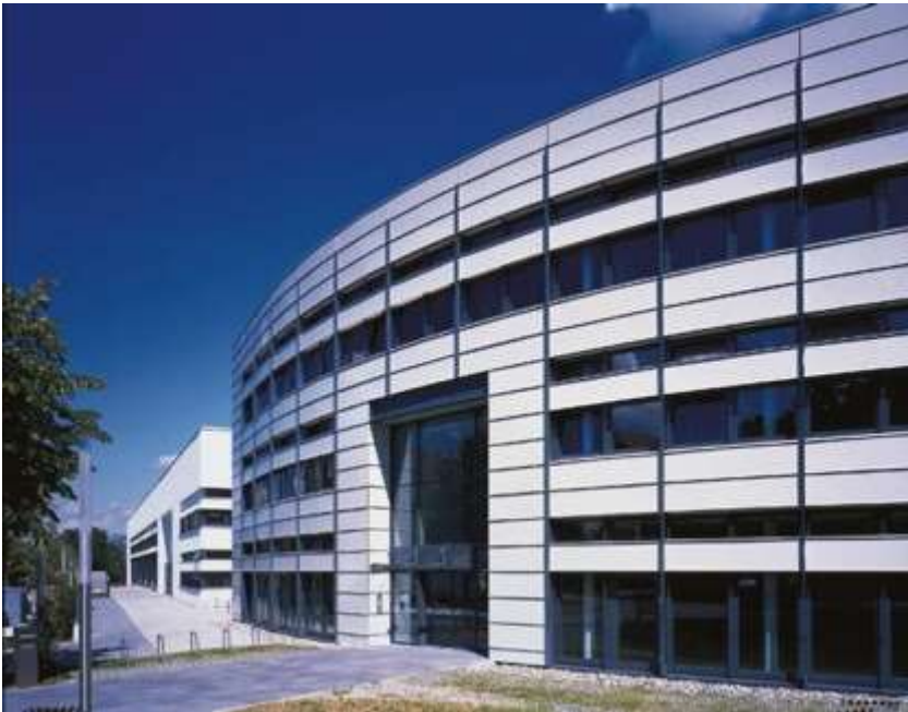
Headquarter of Fraunhofer ISE, Freiburg, Germany
