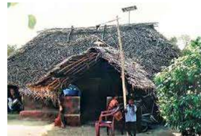
Solar rural house
