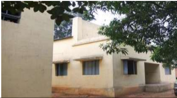
Storage & equipment sheds
